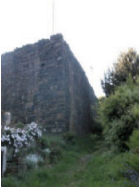
The highest corner of the 18ft wall
