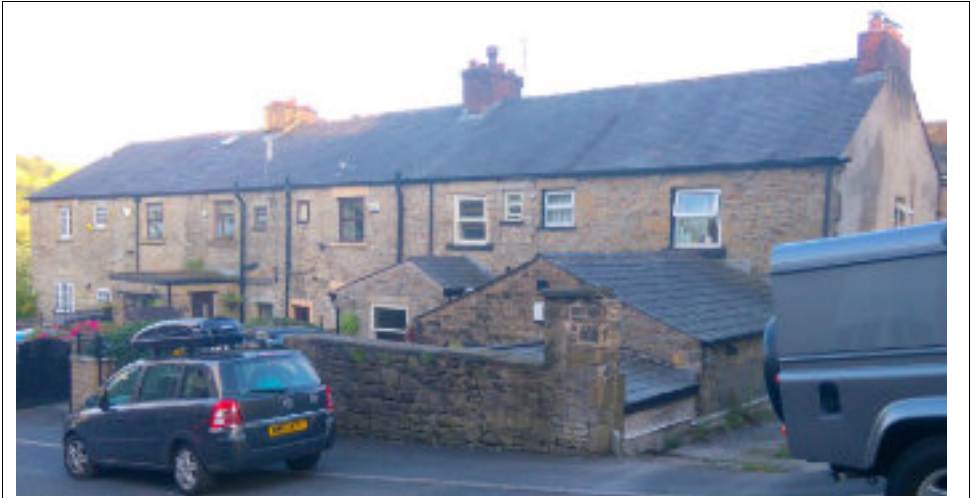
Figure 2: Scotland Place originated as Peel and Yates' cloth drying house. When the Old Ground was abandoned in the 1820s, the drying house's shape lent itself to conversion into a terrace of cottages. This photograph shows the building before the extension was completed in 2008.
