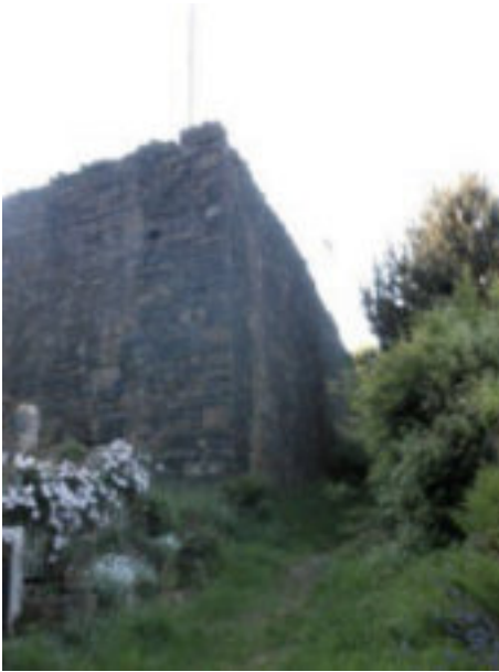
The highest corner of the 18ft wall
