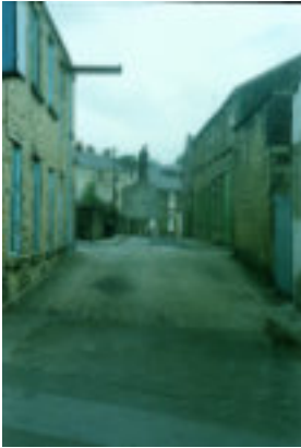
Photo: June 1987 – looking north along Prince Street. Strang's Iron Foundry, by then Metcalfe Bros Ltd, pallet makers, on right.
