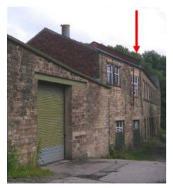
The west face of the mill had a very clear building break, (indicated by the arrow). The portion of the mill to the right of the break was built from a much better quality of stone, quite carefully dressed almost to ashlar standards, with good quality lintels sills and reflecting improvements in quarrying techniques achieved by the time that this section was erected. It probably postdated the 1847 Survey Ordnance map, perhaps comprising a later stage of development.
