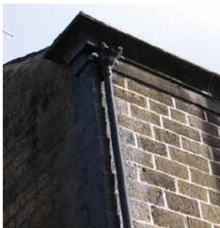
Fig. 79 Watershot masonry and stone gutter on Bury New Road
