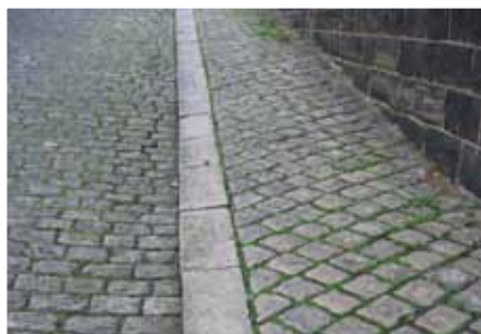
Fig. 58: Well-laid historic setts on Vesta Street
