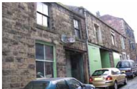
Fig. 34: Little altered workshops on Paradise Street
