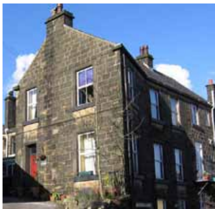
Fig. 37: Changing levels on Milton Street
