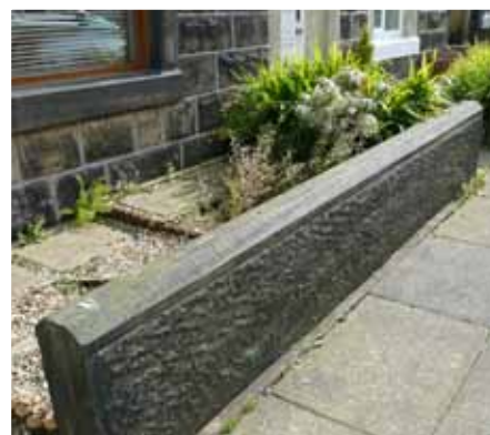
Fig.83. Single-slab stone wall, Major Street
