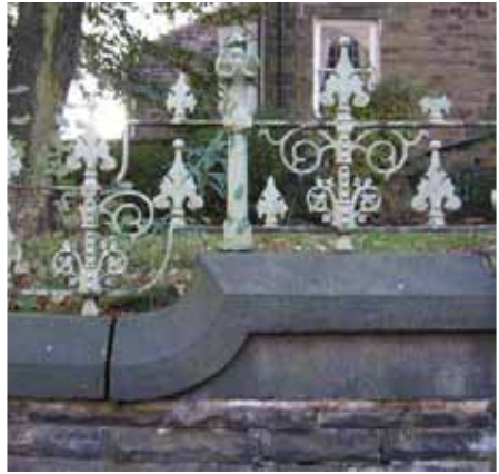
Fig. 71: Ornate railings on Garnett Street
