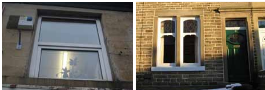
Figs.87 and 88: A modern replacement window on the left. On the right are historic sash windows, on Eliza Street
