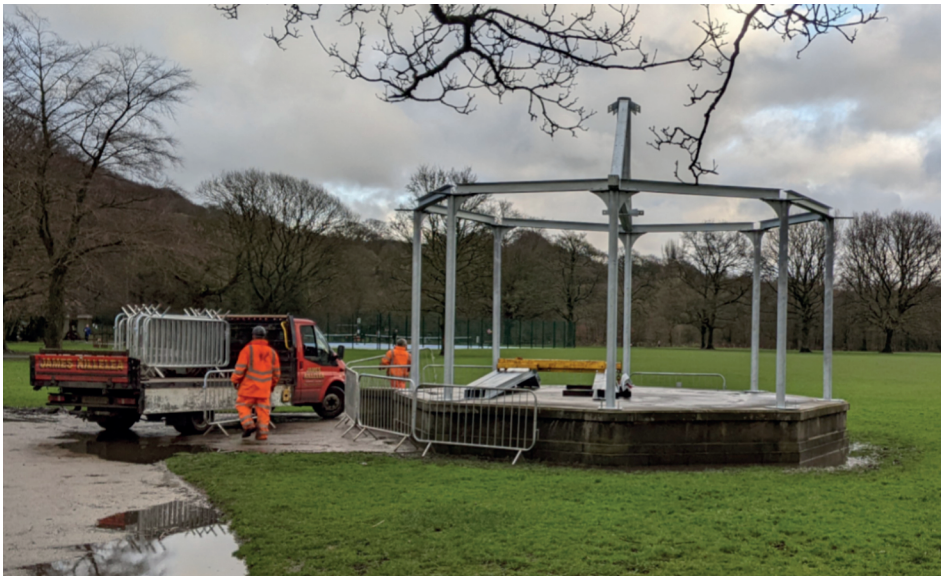
Installation day 14 th February 2022 - Photo by John Leyland
